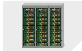
Electric Energy Storage
